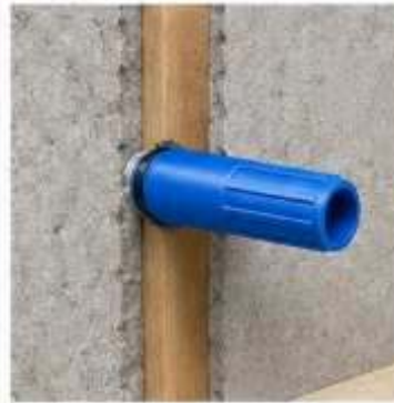
Stub-out fixed in the wall before wall finishing.
